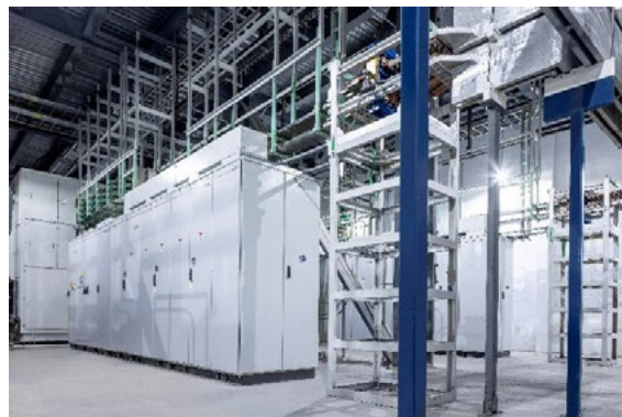
Fig.9 - X-Pact® AURATM installation in the EAF power-feeding room.
