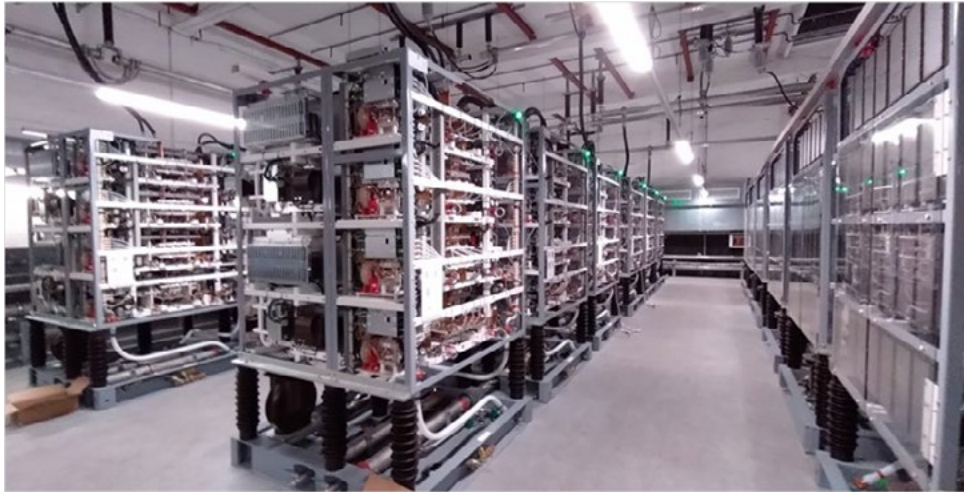
Fig.3 - Photo of the 18 HB towers that interlink the DC bus of the DF converter with the EAF transformer via three arm inductors. Each HB tower contains four power stacks.
