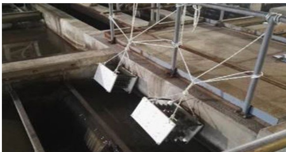
Fig.3 - Illustration of the field exposure of corrosion modules at the Brussels WWTP.
