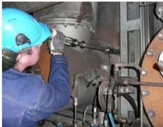
**Fig.6** - Installation of a high-velocity lance as part of a REBOX HLL system at Outokumpu's plant at Tornio, Finland.
