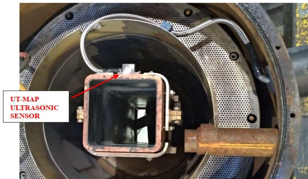
**Fig.2** - Installation of Ergolines' ultrasonic sensor in the water jacket for Ultrasonic Thermal MAPing (UT-MAP).
