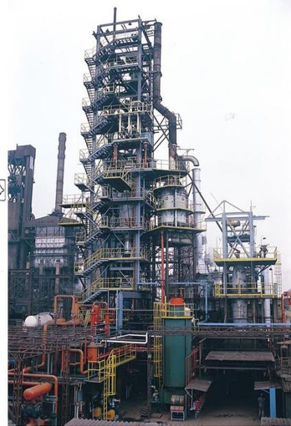
Fig. 4 – HYL Pilot Plant tests campaigns with  $\geq 90\%$  H<sub>2</sub>
