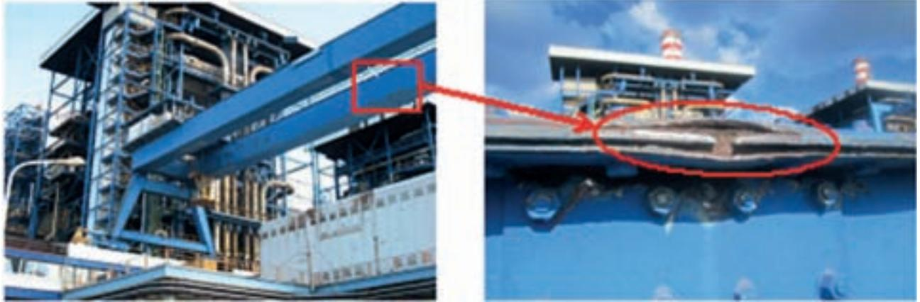
**Fig. 3 – Gantry crane with indication of the joint affected by crevice.**
