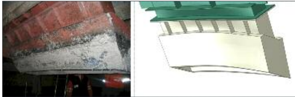
FIG. 5 Bulging of the snout-end rear side is well reproduced by the model.
