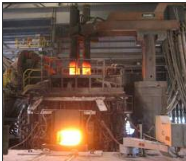
FIG. 1 Jacksonville electric arc furnace.
