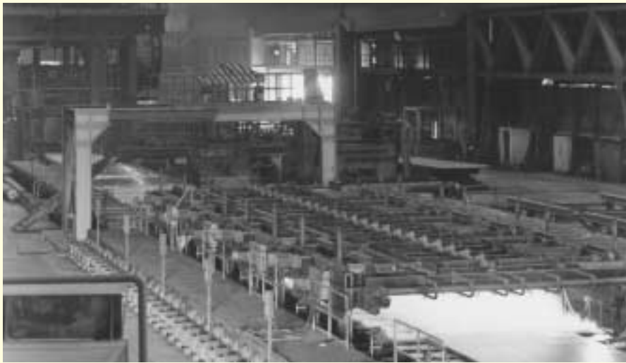
Figure 6: MULPIC System at the Dillingen Plate Mill.
