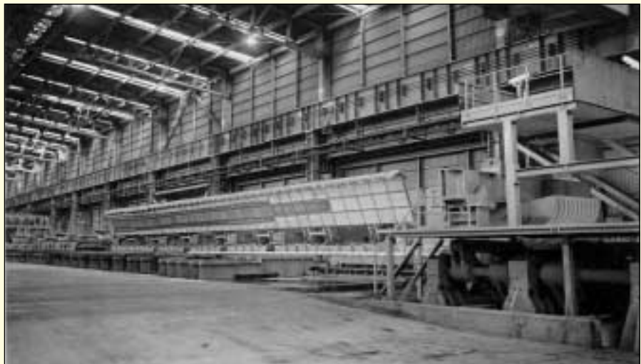
Figure 1: VAI ENCOPANEL System Installed at China Steel's No. 2 Mill.
