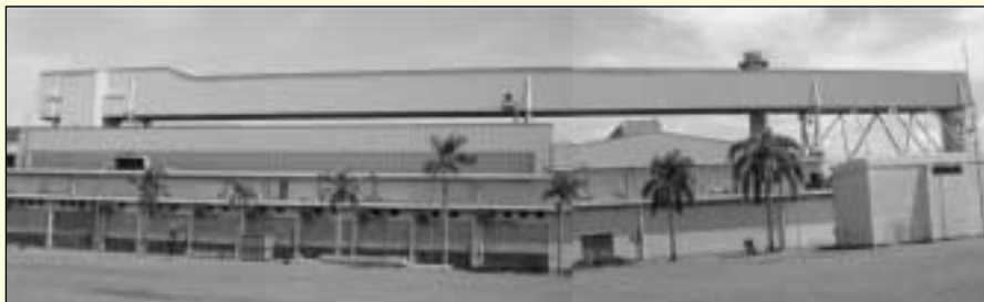
Figure 3: Looper Installed on the Roof at Krakatau Steel, Indonesia.
