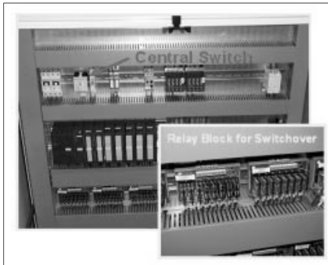
Figure 3: Automation Switch-Over Between Old and New Systems (Selection of active system by one central switch).
