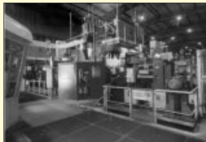
Fig. 4 – Flash Butt Welder 21 (Front View, Exit Section), Sollac Mardyck, France.
