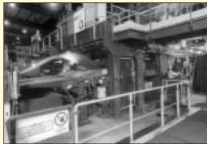
Fig. 3 – Flash Butt Welder 21 (Front View, Entry Section), Sollac Mardyck, France.
