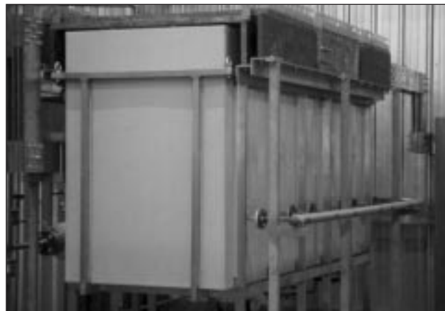
Fig. 12 – Impianto pilota processo pirometallurgico c/o AST. Fig. 12 – Pilot plant of pyrometallurgical process c/o AST, Terni.
